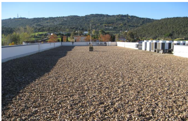
Roof of the Spanish building
